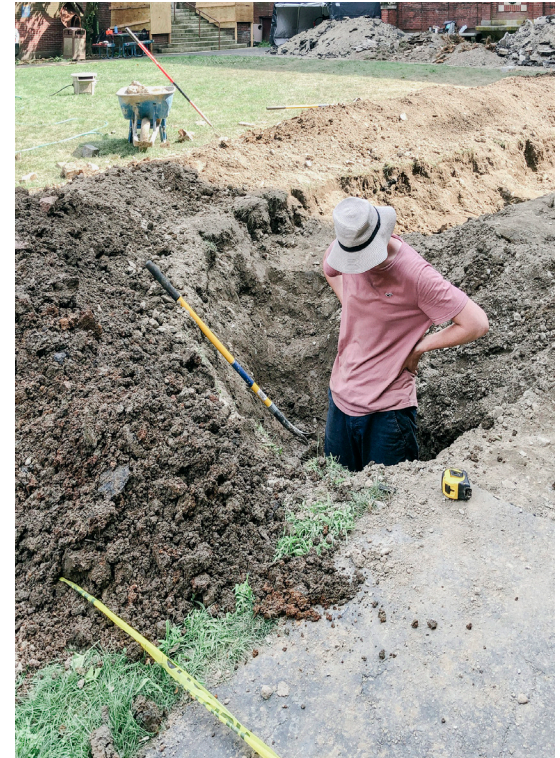
Left: The team digs a four-foot deep trench by hand.
