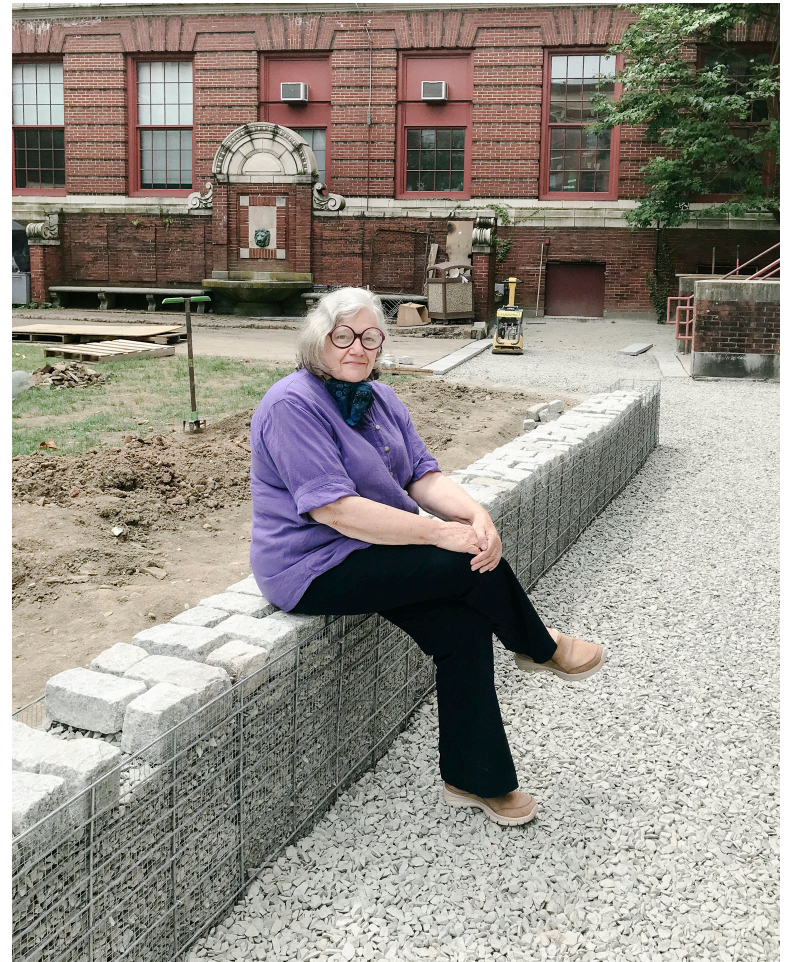
Meg Hickey, our structural engineer, approves of our wall.
